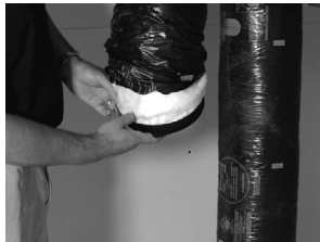
Insert insulation inside the double collar.
