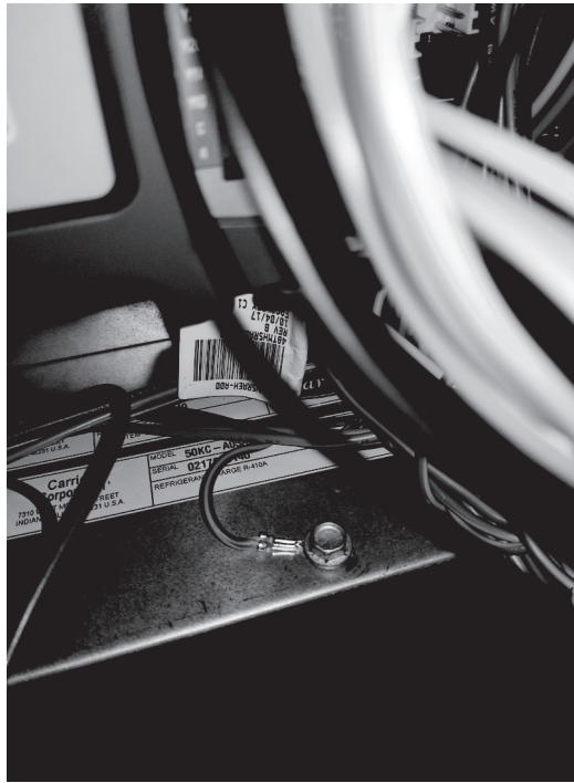
Fig. 20 — Connect Ground Wire From Controller
