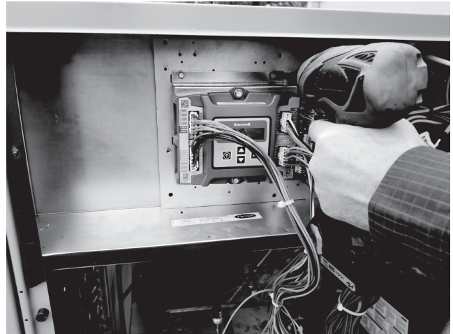
Fig. 15 – Mount Controller Assembly in Unit Control Box
