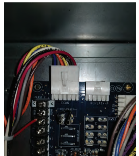
Fig. 22 - Harness Detail
